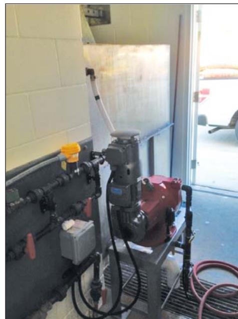
On-Site Lime Mixing and Dosing System
